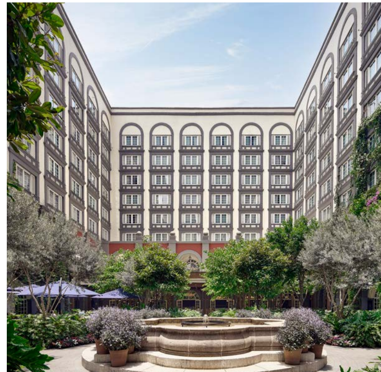
Four Seasons Hotel Mexico City courtyard
